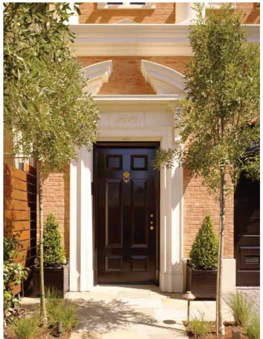
The front door, with a broken pediment as the focal point, was inspired by the George F. Baker house in New York City.
