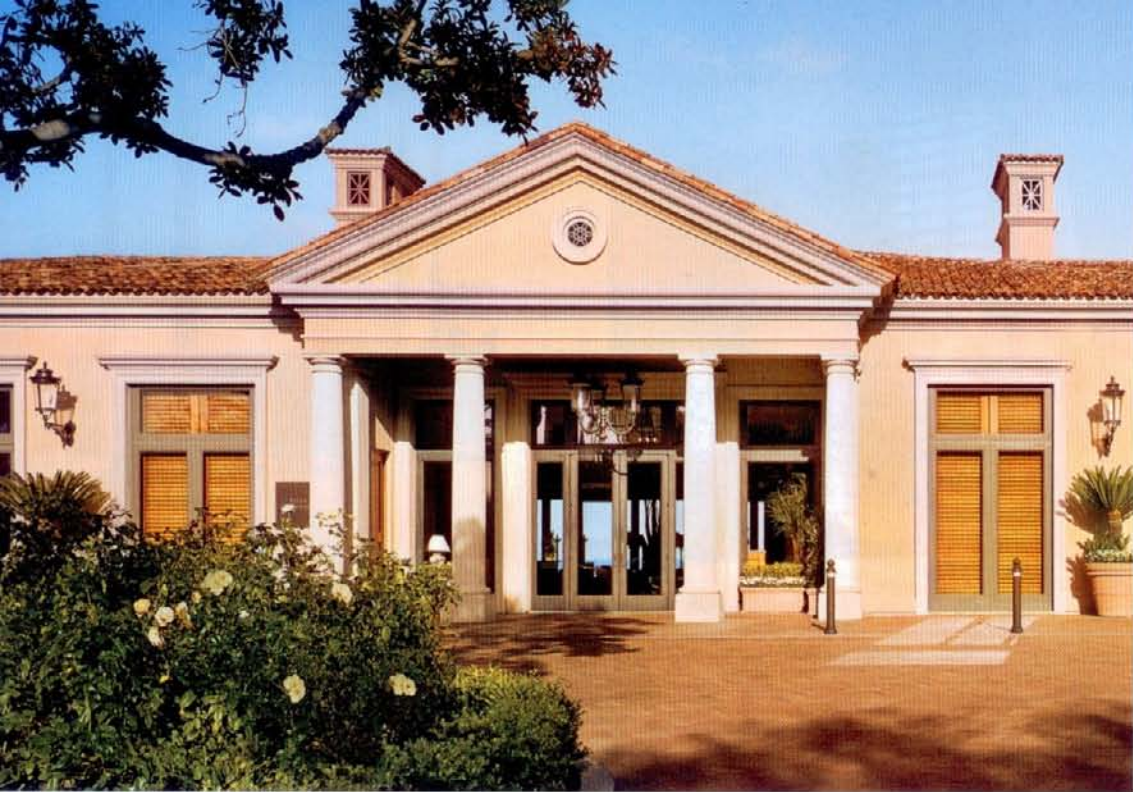
LEFT: A portico of the Tuscan order identifies the entrance to the Villa Clubhouse, whose amenities are reserved for villa guests. The hotel's grounds were planned by Burton Landscape Architecture Studio. BELOW: The clubhouse pool.
